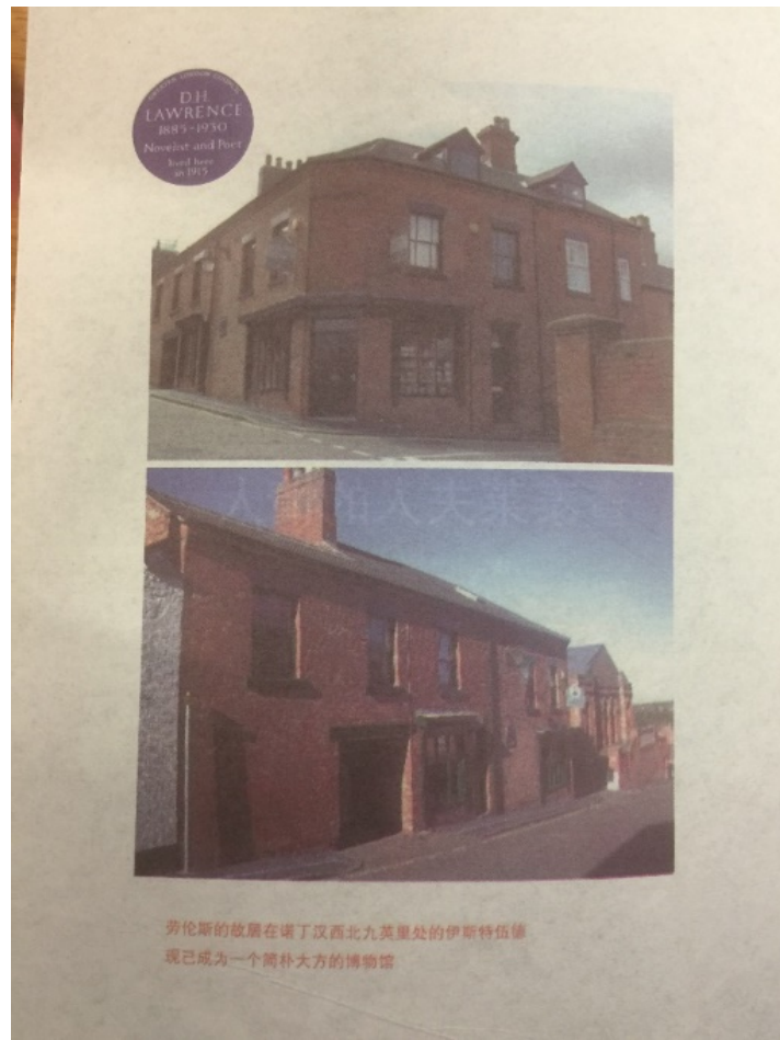
6.3-9 Lawrence's former residence
