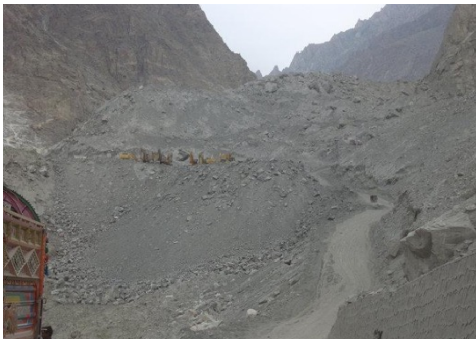
Figure 44. Dirt road carved through the landslide debris, 2011.
