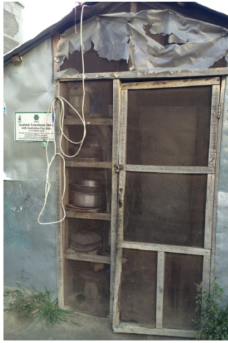
Perforated steel sheet used in front for ventilation, with items placed in shelves behind it.
