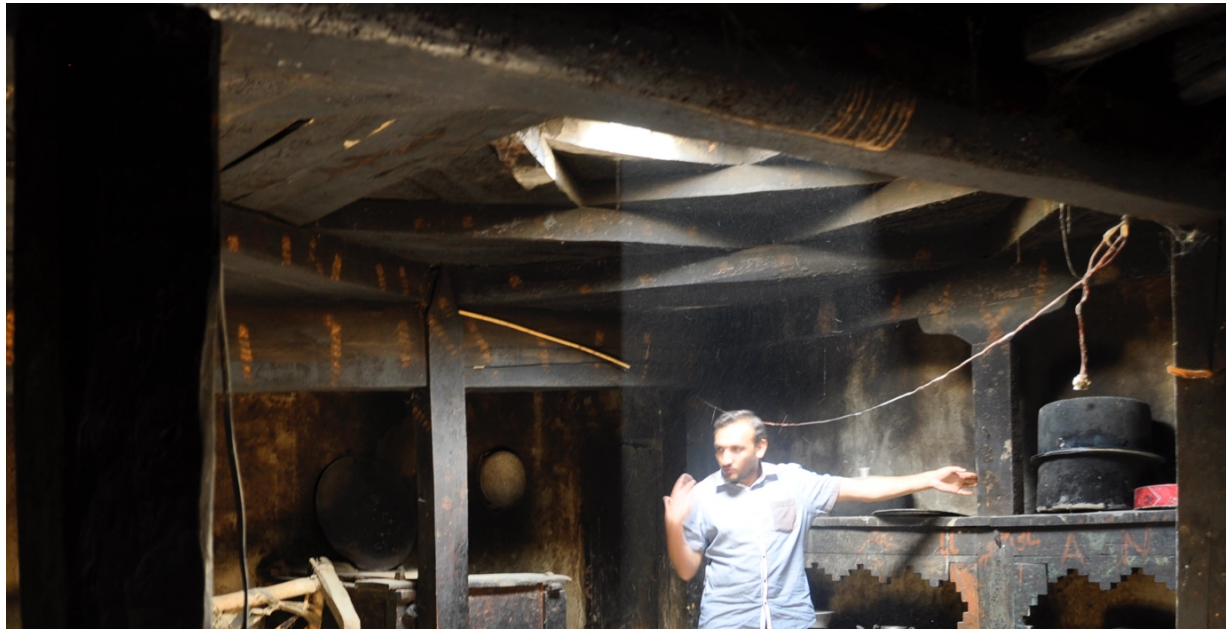
Figure 40. Stacked wooden octagonal roof ending in a square skylight – Wakhi House.
