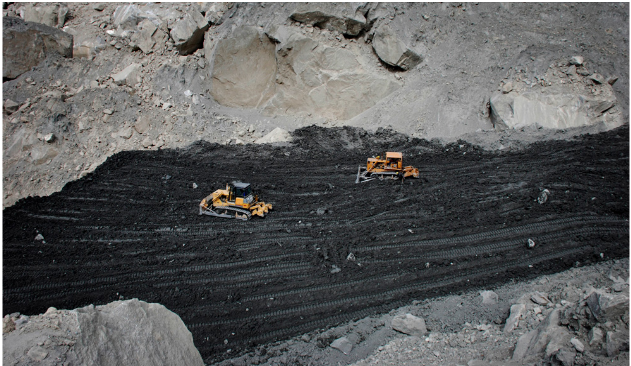
Figure 8. FWO preparing the debris surface for construction of spillway
