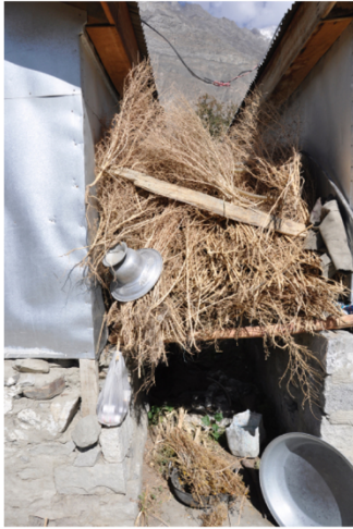
Grass is held with wooden support fixed between two shelter units.
