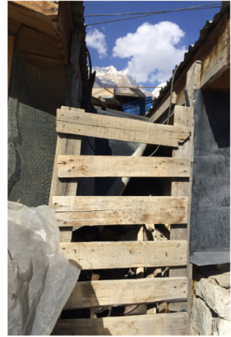
Horizontal wooden planks nailed to vertical posts to secure items stored between shelters
