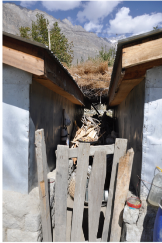
Wooden planks installed vertically to secure items stored between shelters
