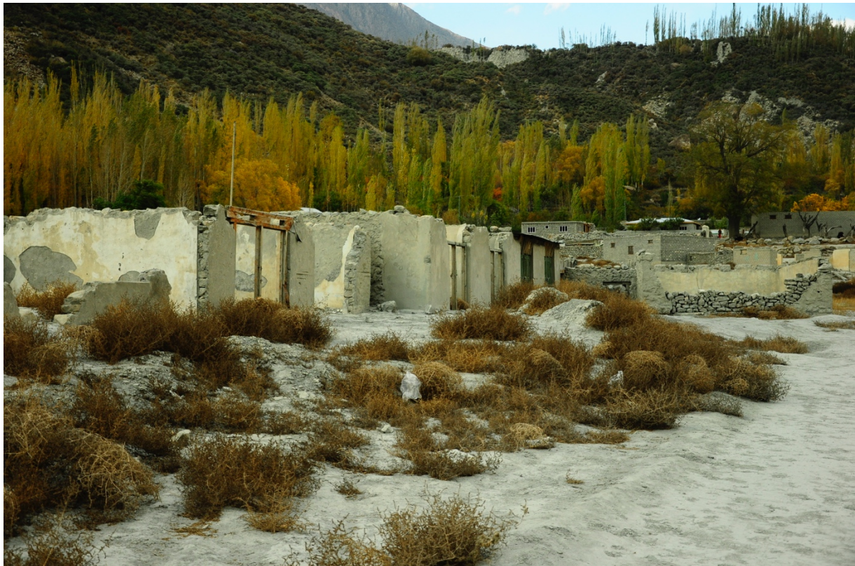
Figure 7. The silt laden scapes in Gulmit after the lake water receded in 2014.
