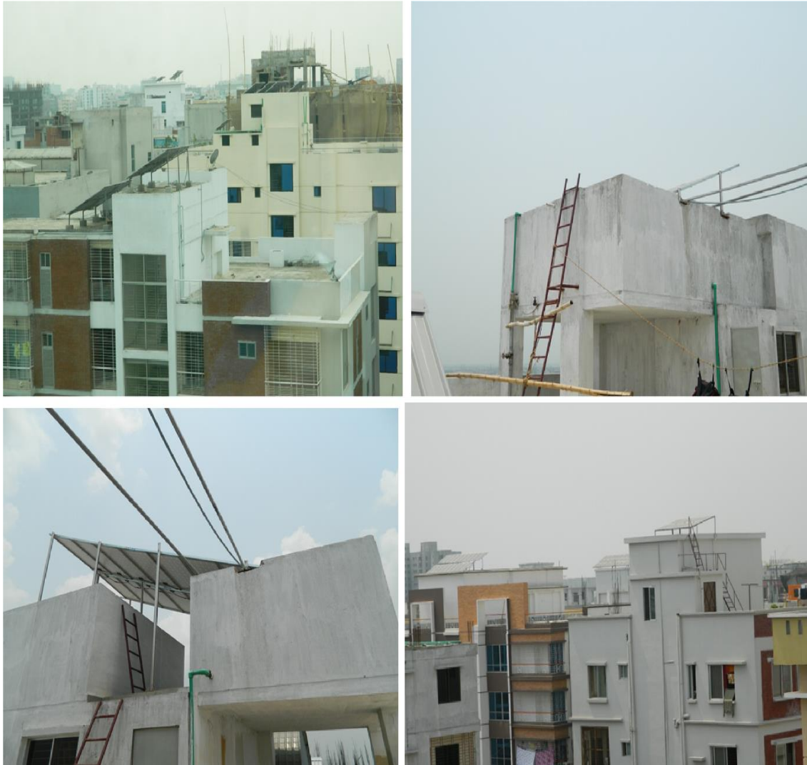
Figure 8:8 Solar panels on rooftops
