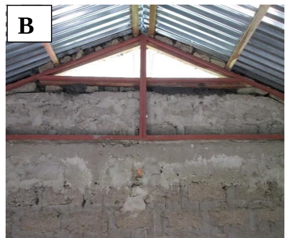
Fig. 2.2: RooPfs house and the gable window: A) RooPfs house B) close-up of screened gable window
