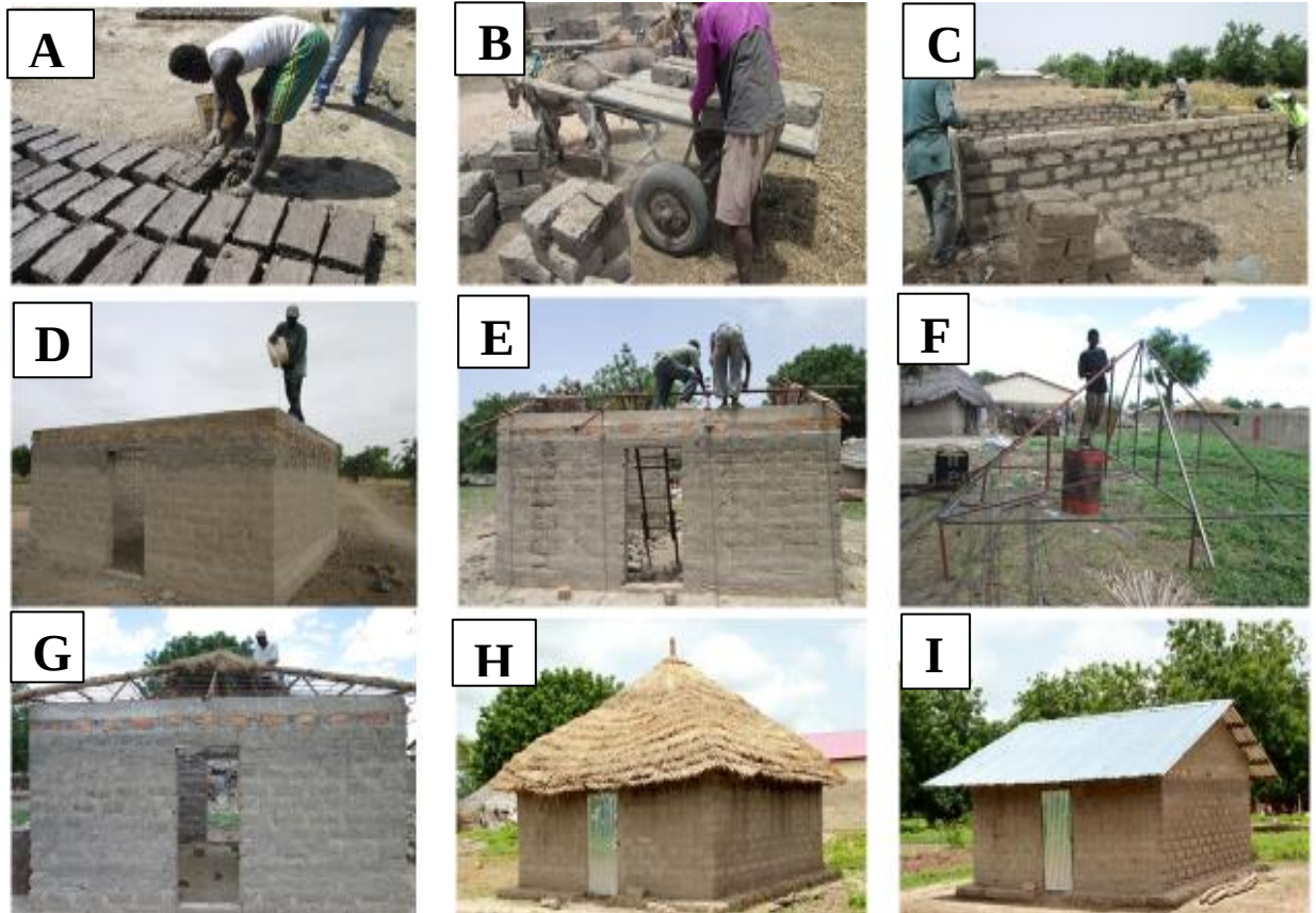
Fig. 2.3: Experimental houses under construction: A) mud blocks being sun dried, B) block transportation, C) wall construction, D) wetting concrete lining, E) attaching wood to metal frame, F) assembling metal roof frame, G) putting thatch on roof frame, H) complete thatch roofed house, I) complete metal roofed house
