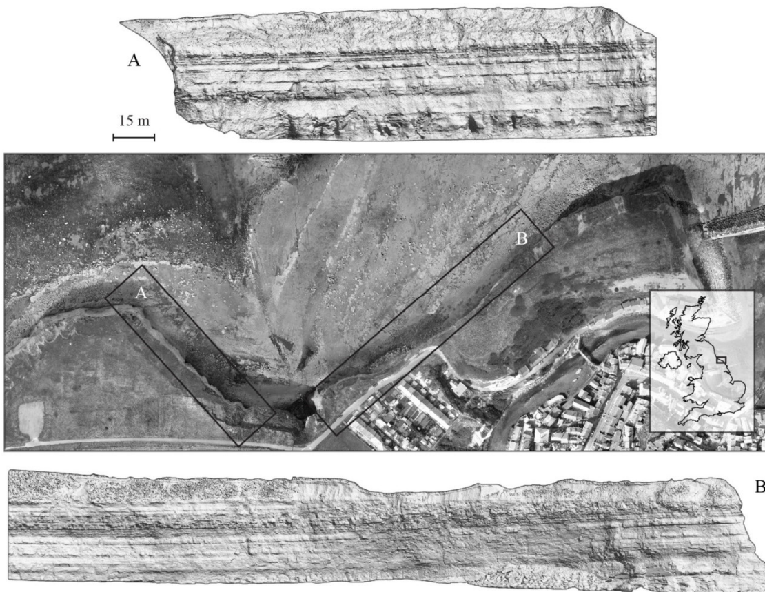
Figure 2. Aerial photo of the coastal rock slopes at Staithes, North Yorkshire. The cliffs are divided into Sites A and B to account for the changing aspect of the coastline.
