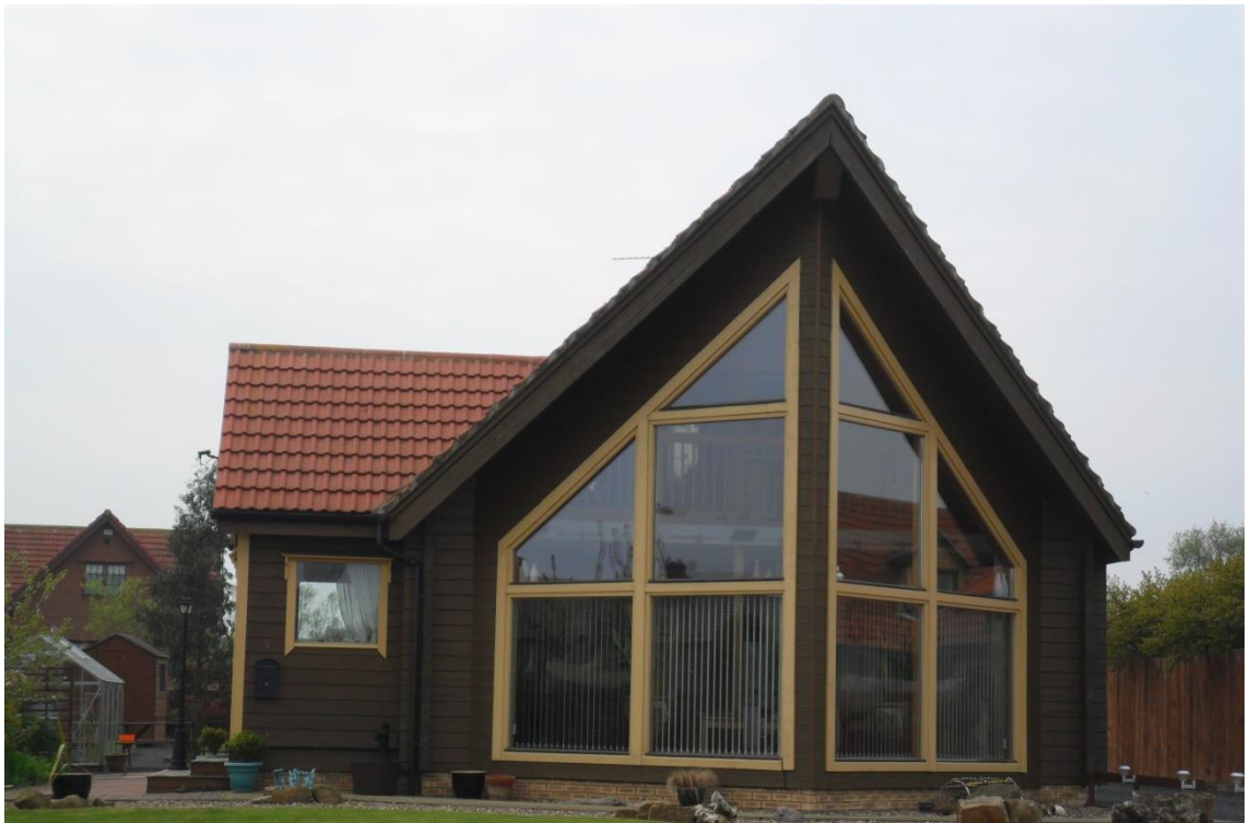
Figure 6.3: Scandinavian style housing development in Hadston
