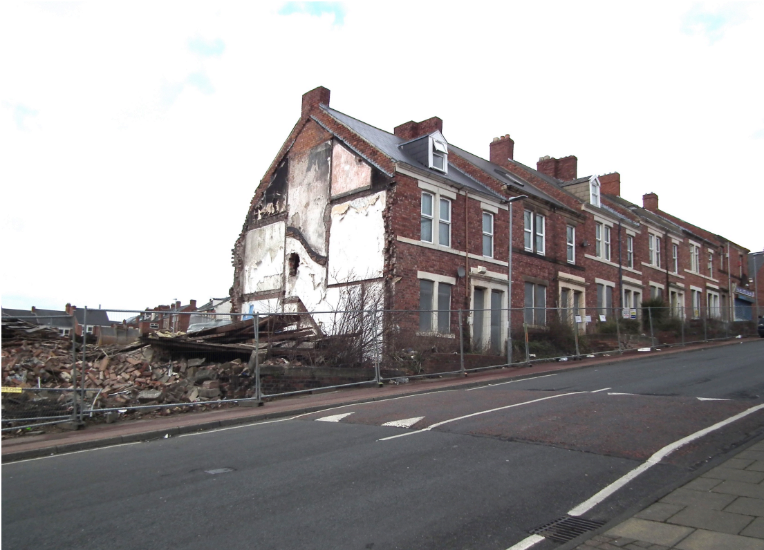
Dunsmuir Grove during demolition, March 2016. Source: author
