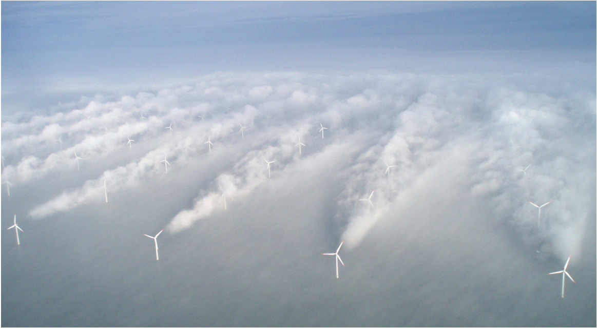
Figure 1.7 Wake effects at the Horn Rev wind farm [15]
