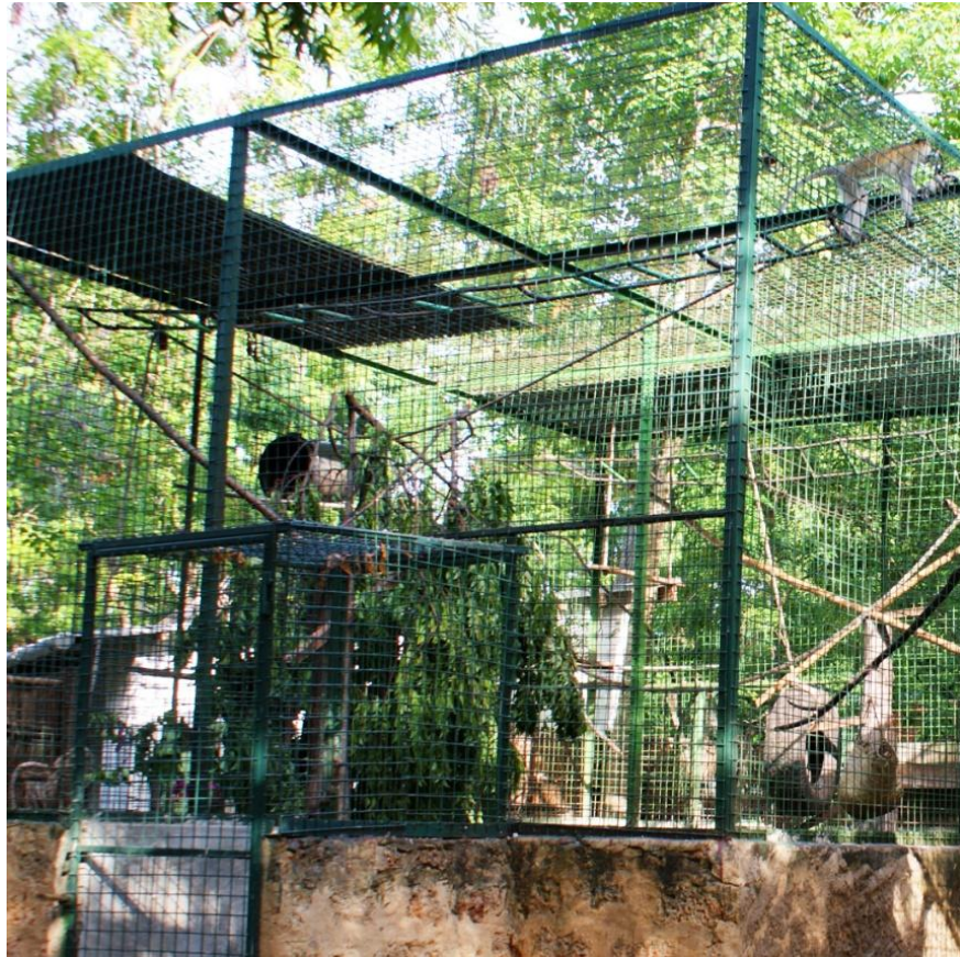
Figure A1.4 An example of a canopy bridge installed within a pre-release enclosure.
