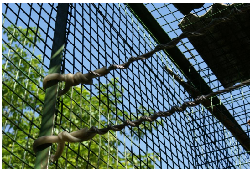
Figure A1.6 An example of insulation between the training electricity cable and the metal enclosure.
