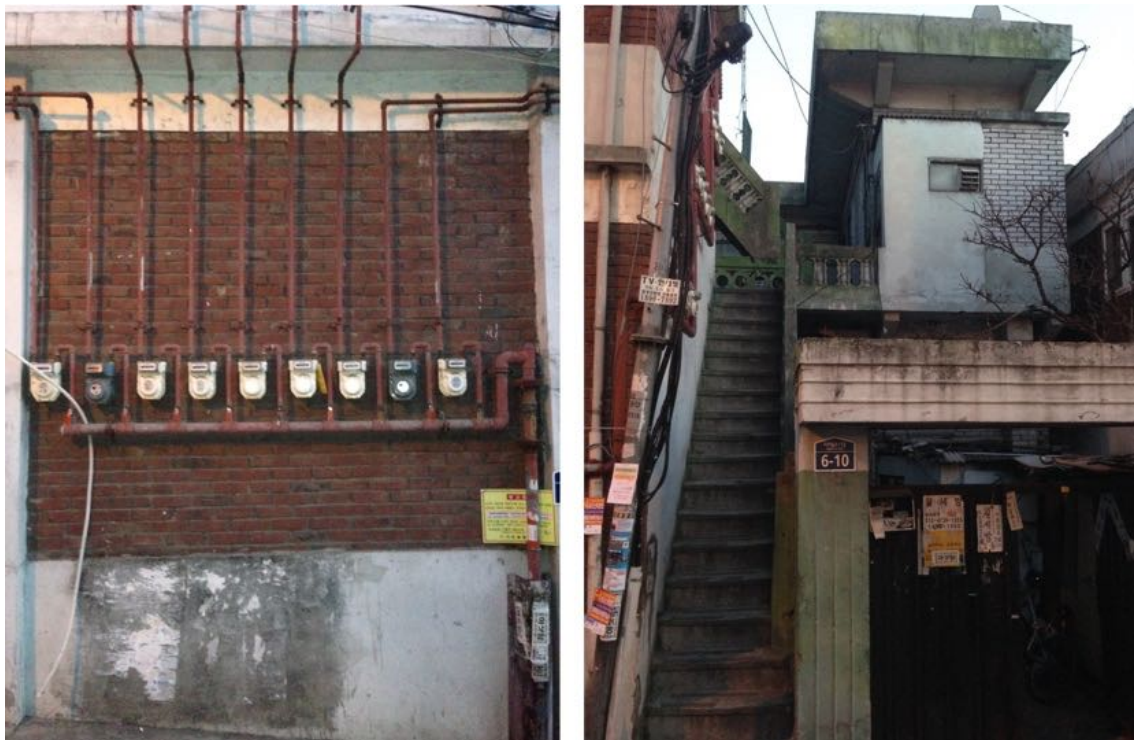
Figure 5.5 Old houses in SDIC2, composed of tiny rooms to rent.
