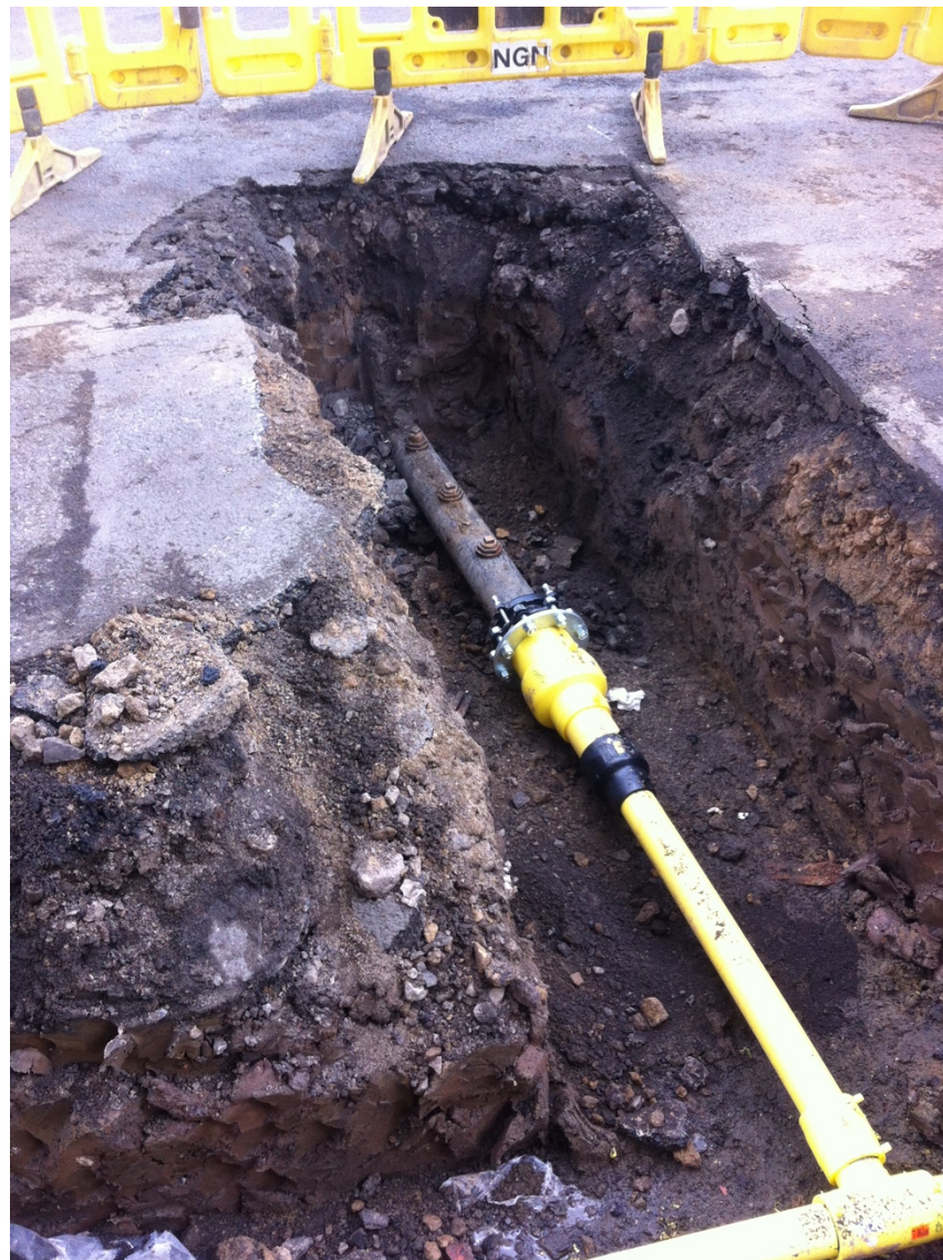
Figure 18 - Photograph of a distribution pipe in Middlesbrough, 2015
