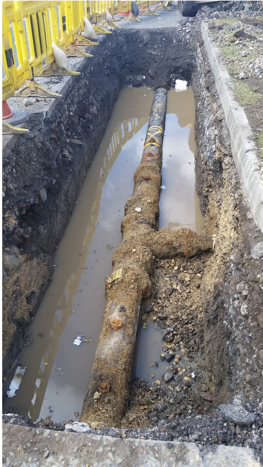
Photograph of excavated cast iron medium-pressure gas main, Neville's Cross, Durham (2016)
