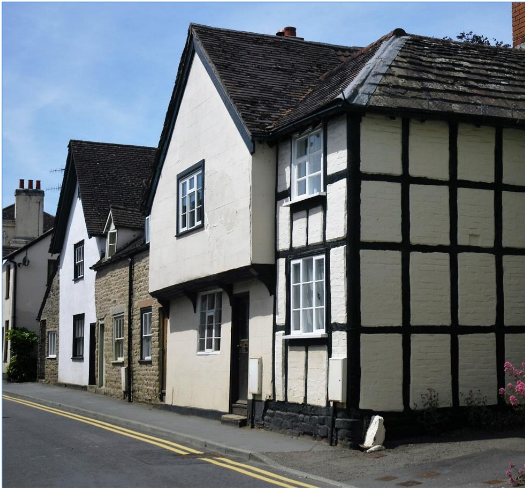
Figure 51. 15C timber-framed hall-house occupying Nos 36-38 Duke Street (TA, 2016).
