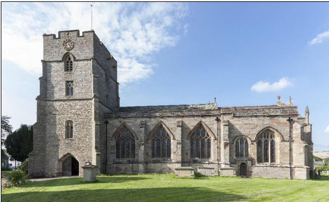
Figure 4. The Church of St Andrew, Presteigne – looking towards the south elevation (RCAHMW, 2016).
