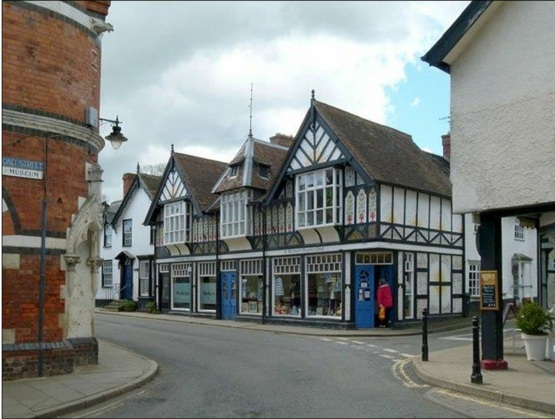
Figure 34. The intersection of High Street and Broad Street, with Hereford Street to the left and Green End to the right (© Copyright Alan Murray-Rust, 2016). The building in the centre of the picture is Radnor House which has a 1890s Arts and Crafts influenced façade, possibly overlaying an earlier structure. The white building to its left dates from 1463 and is an example of a hall and cross-wing house. The red brick building on the left of the picture is the Victorian Italianate Market Hall and Assembly Rooms. The jettied building on the right of the picture is of 16C origin.
