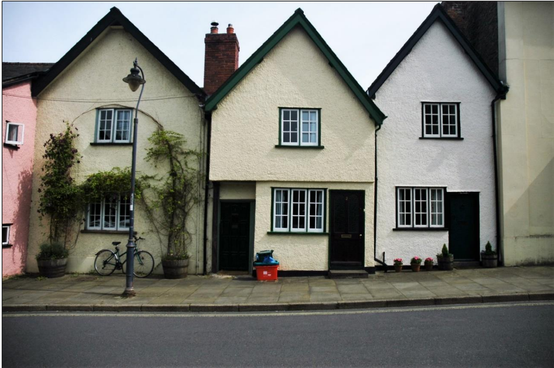
Figure 83. Oak Villas, Broad Street, Presteigne. A cruck-framed hall-house (TA, 2015).
