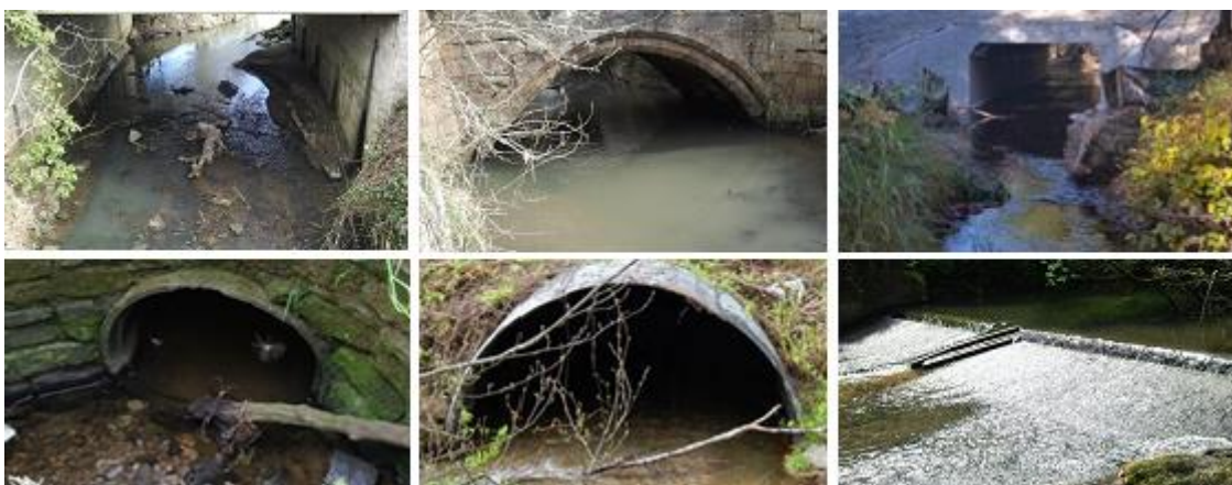
Figure 2.5: Examples of structures near which sections were surveyed for fish community composition. Top row: left: box bridge; middle: arched bridge; right: box culvert; bottom row: left: pipe culvert; middle: arched culvert; right: vertical weir, preceded by a ramp.
