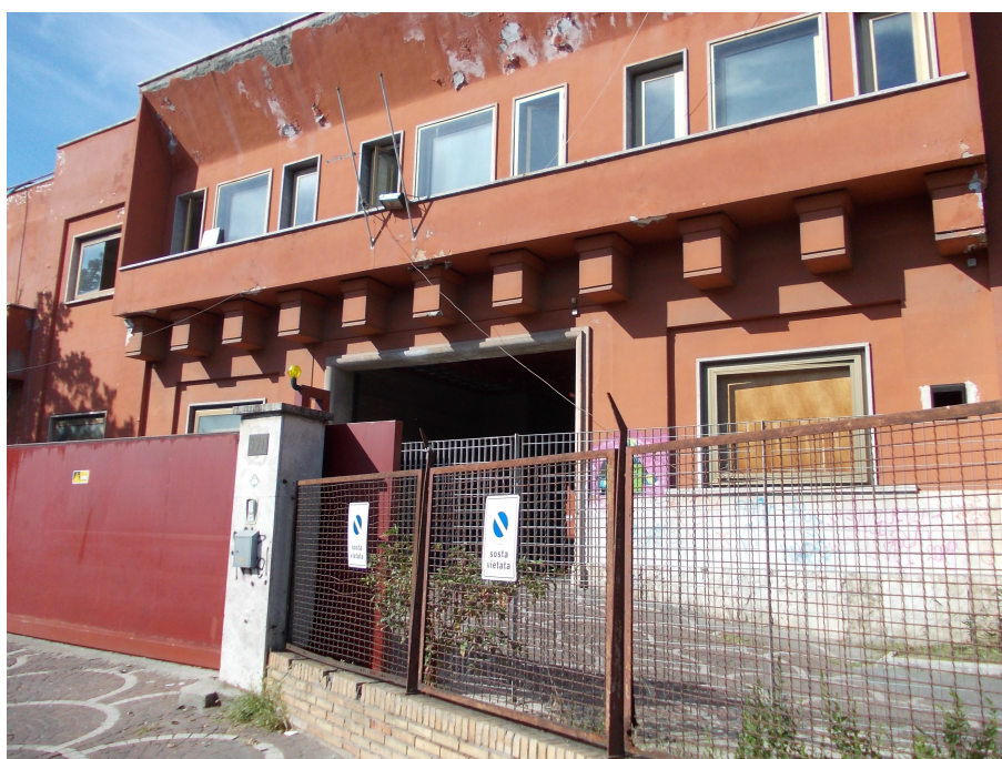
Figure 5.1 – The entrance gate of the Cartiera centre
