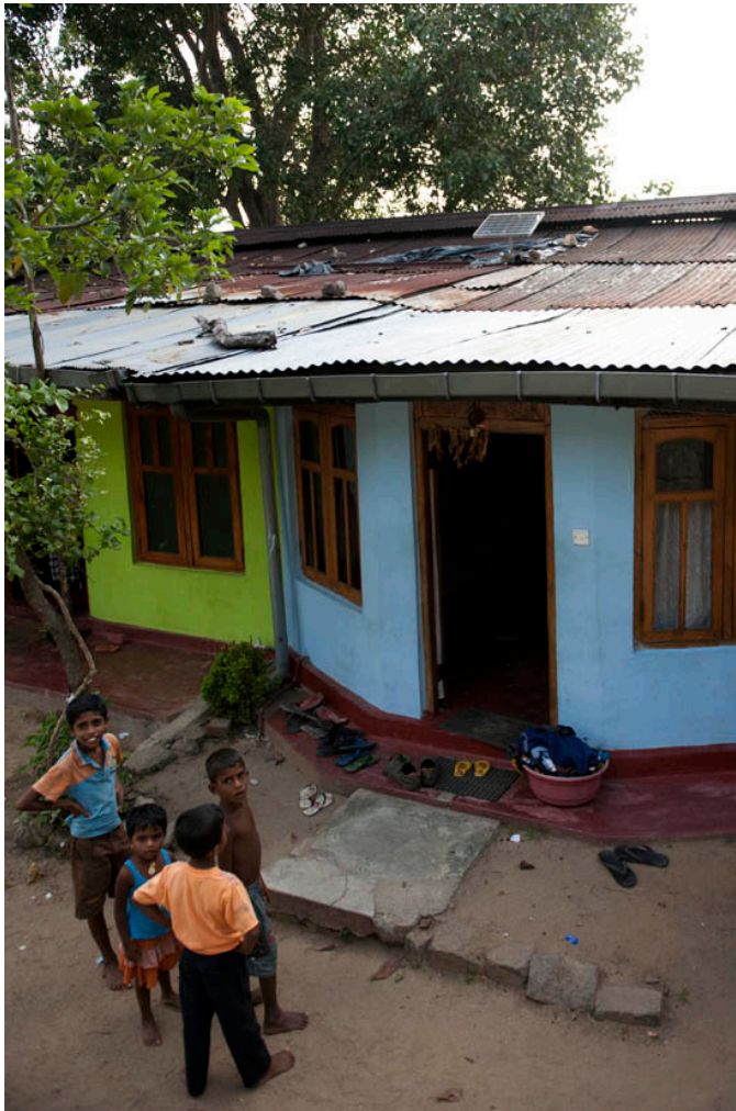
Figure 4-5: Solar Home System installation, Monoragala, Sri Lanka
