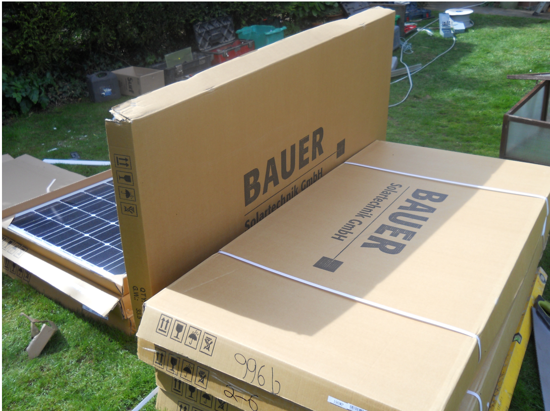
Figure 4-2: Solar installation at Peter and Anne's home panels and tools
