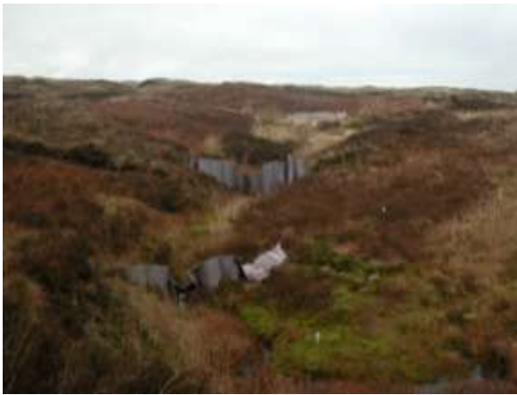
e) Gully blocked, seeded and limed (SL.B-G)
