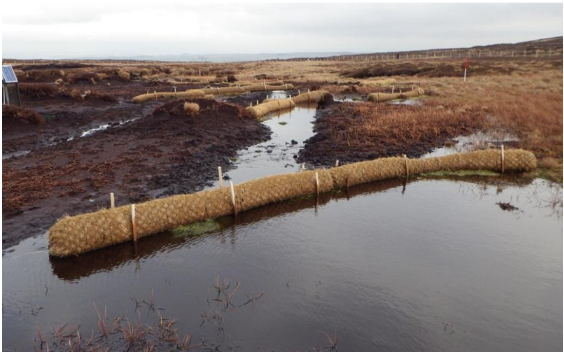
Figure 8.3 – Examples of eroded peat being trapped by (a) vegetation at the margin of bare peat (b) coir rolls.
