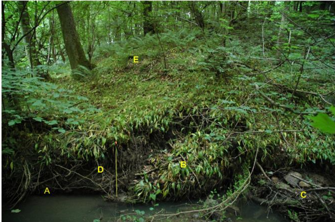
Figure 5.4-Initial photography providing a base line for change. A – Bank undercutting. B – Bank collapse. C – Debris blocking the stream. D – Root system. E – Steep forest with curved trees. The meter rule by the root system, provides information on scale.
