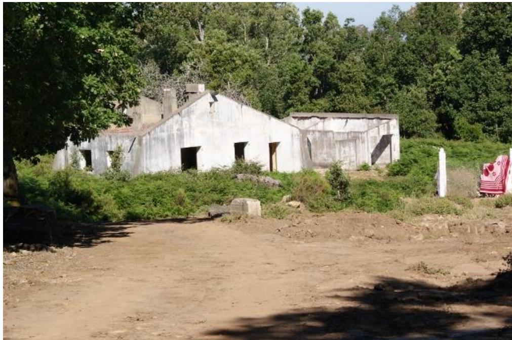
Figure 3.1. The now derelict Spanish Civil Guard and Forestry Headquarters in Bouhachem
