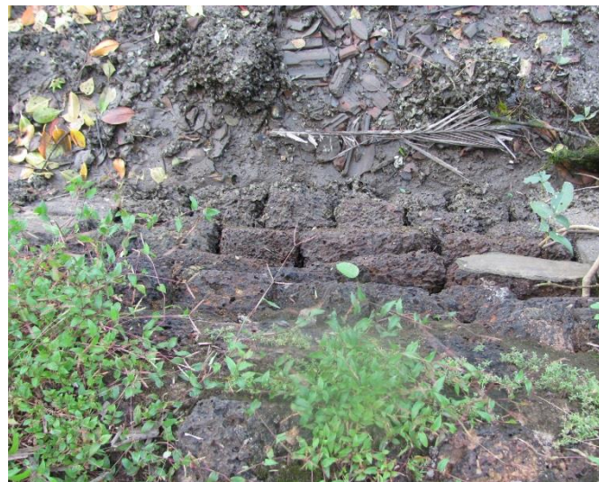
Plate 5e: Laterite revetment of channel bank north of church
