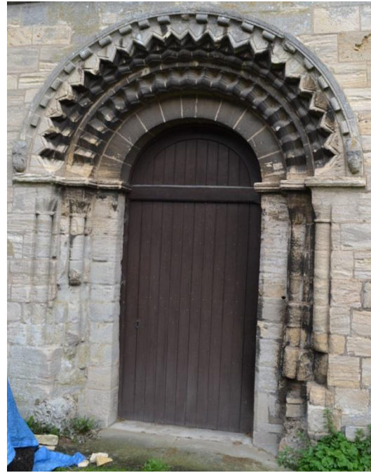
Fig. 4c. Nave west doorway, St Swithun, Leonard Stanley, Gloucestershire.
