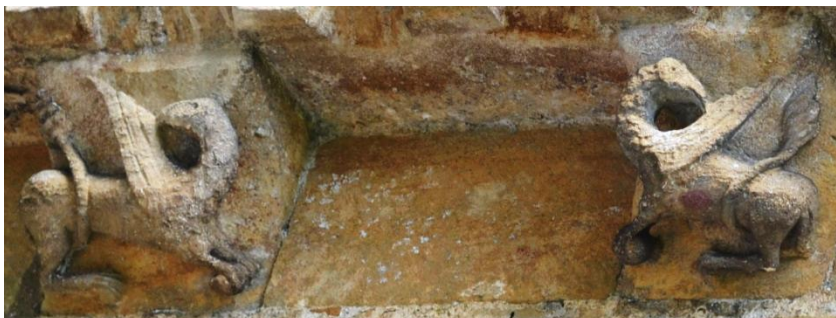
Fig. 24e. Corbels, south nave exterior, St John the Evangelist, Elkstone, Gloucestershire.
