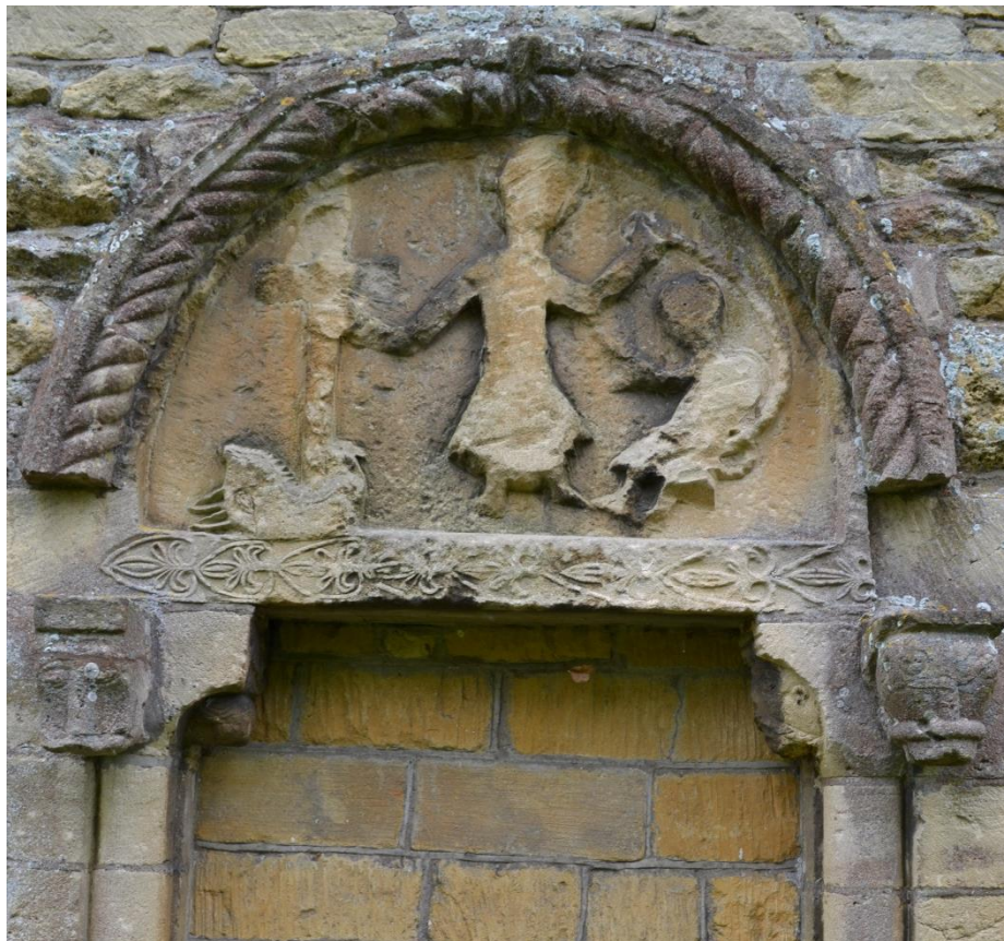
Fig. 3k. Nave north doorway (blocked), St John the Baptist, Beckford, Worcestershire.
