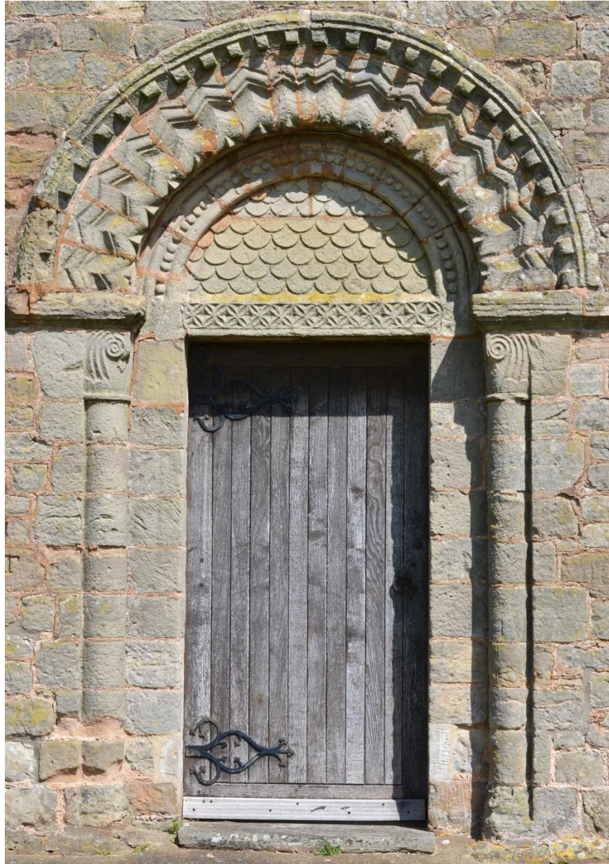
Fig. 5h. Nave south doorway, St John the Evangelist, Pauntley, Gloucestershire.
