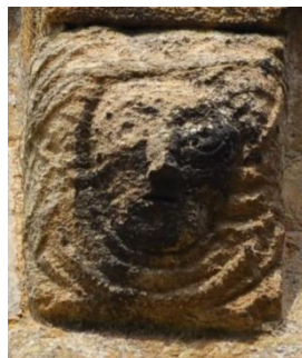
Fig. 14d. Corbel, south-east chancel exterior, St Peter, Siddington, Gloucestershire.
