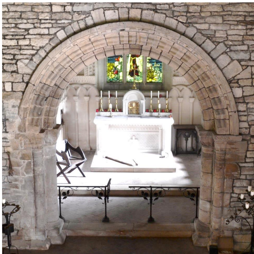
Fig. 3h. Chancel arch, St James, Postlip, Gloucestershire.
