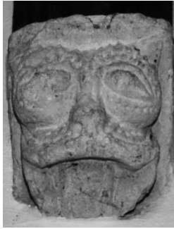
Fig. 19d (left). Reset corbels, nave interior, St Peter, Windrush, Gloucestershire.
