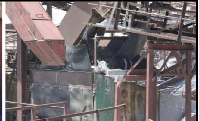
Material reaches the processor and is crushed and screened
