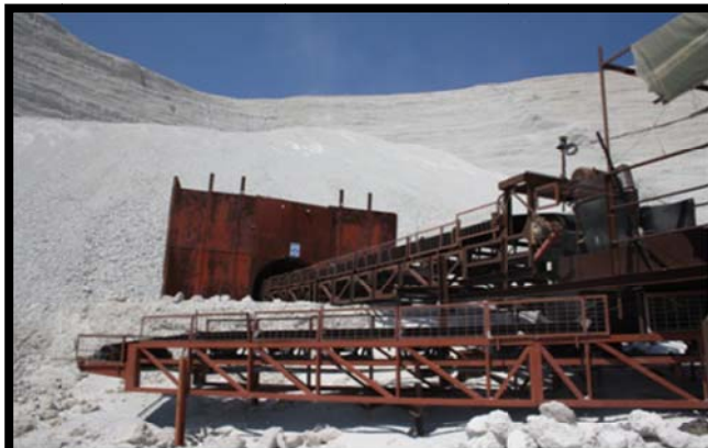
Pumice is dug from the wall and pushed by a front loader onto the roof of a tunnel
