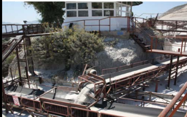
Processed material travels by conveyor belt either to a stockpile, or out to sea...
