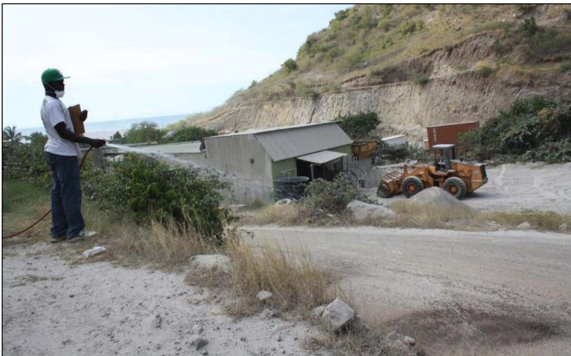
Figure 6.20 Spraying water with a hose to minimise the dust from the road from becoming re-suspended at Little Bay, Montserrat. Note the worker is wearing his respiratory protection on his chin.
