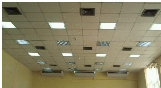
Figure 4.7 Classroom Ceiling in Distance-learning Classrooms in KSU
