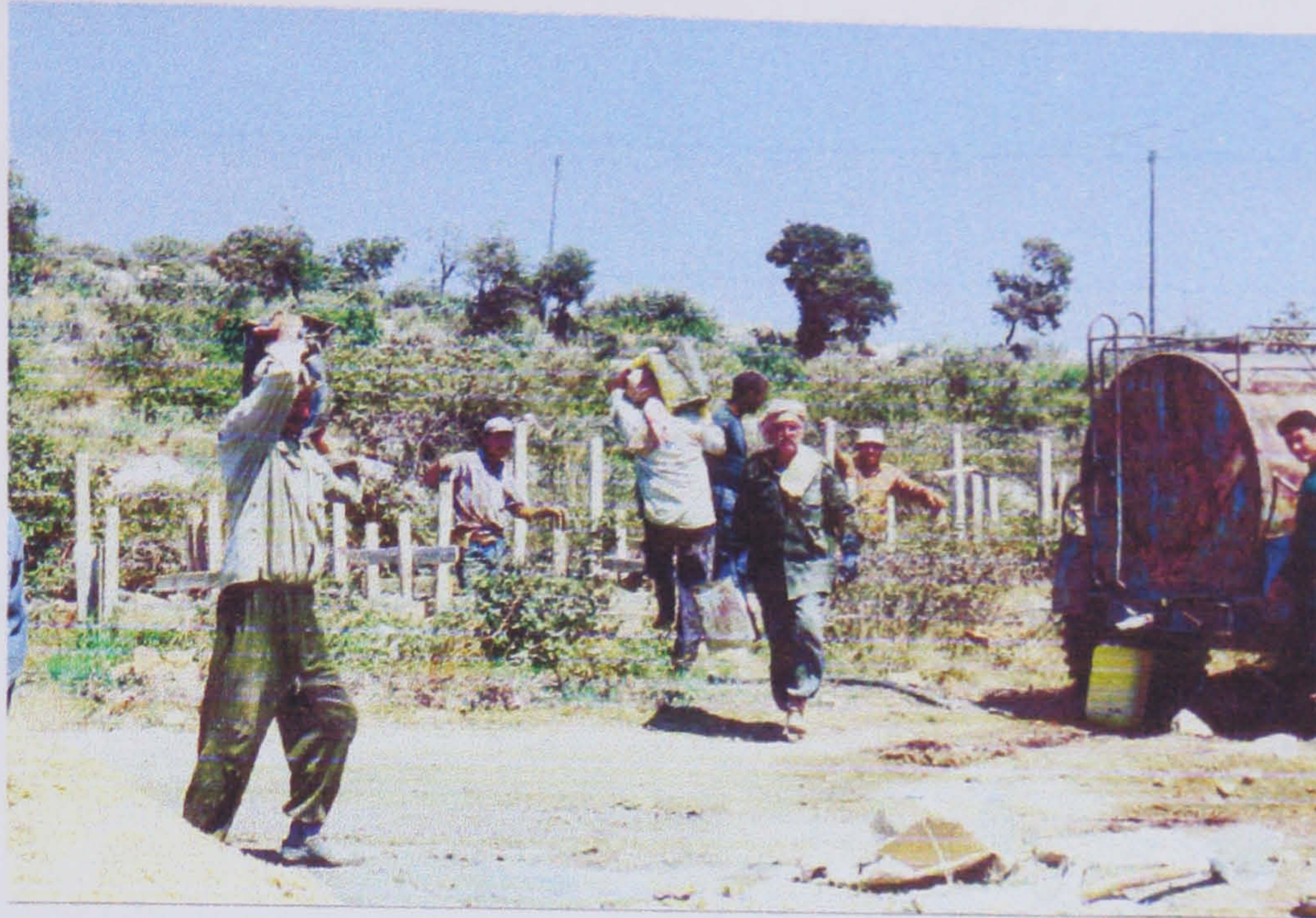
Men at work on a CHF site in Wadi Khaled
