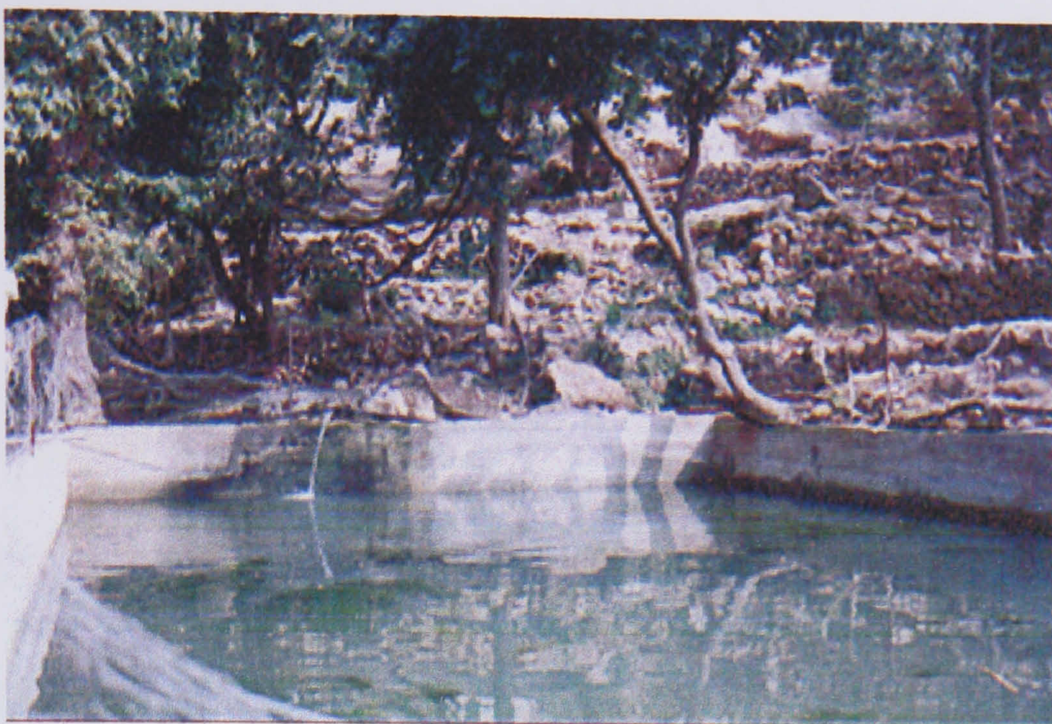
Mercy Corp's water reservoir in Bajaa'
