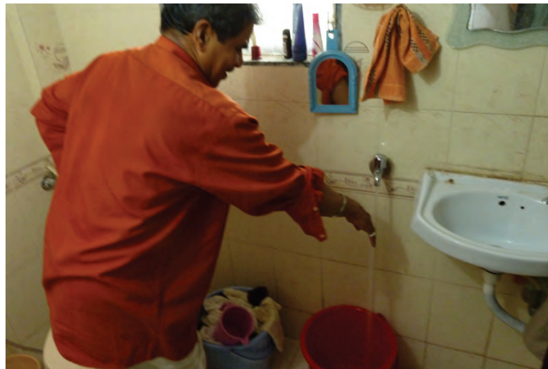
Figure 7.8: User testing the temperature of the SHW in order to soak clothes for washing purposes, Thane.
