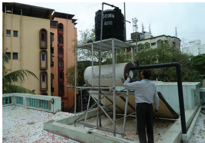
Figure 6.11: Dealer of SHW systems performing a site visit, Thane.
