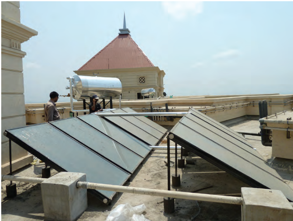
Figures 6.24: SHW at the Gemini Tower (Hiranandani Meadows). The system is composed of 2 tanks and 11 collectors per tank. With 1,300 litres per tank, the system provides 2,600 litres of hot water every day. The tower has 27 stories and 104 flats. The system provides 25 litres per flat.
