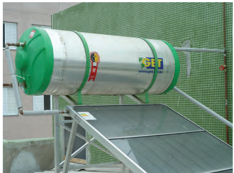
Figures 6.5 and 6.6: Energy label for SHW systems developed by INMETRO (INMETRO, 2013) and SHW system based on flat plate collector technology in social housing in Cubatao, Greater São Paulo Brazil. Note the PROCEL Seal on the tank (red, yellow and black) and INMETRO's sticker (top left corner of the collector), as part of the Brazilian Labelling Programme.
