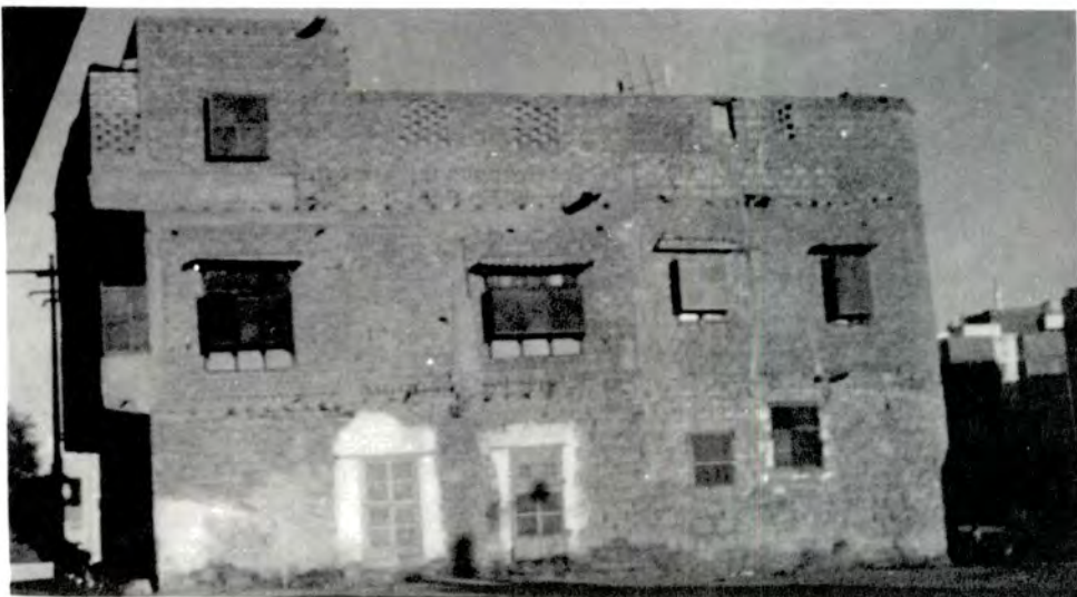
Plate 1.3 The ground floor of this building is constructed from stone and the first floor from concrete.
