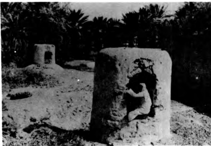
Plate 2.6 Openings along the subterranean canal used for cleaning purposes.
