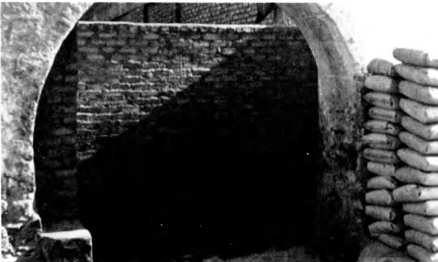
Plate 2.5 One of the Ayn Az-Zarqa watering places with recently bricked-up stairs. Its taps can be used for ablution, as it is near Abo-Bakr mosque.
