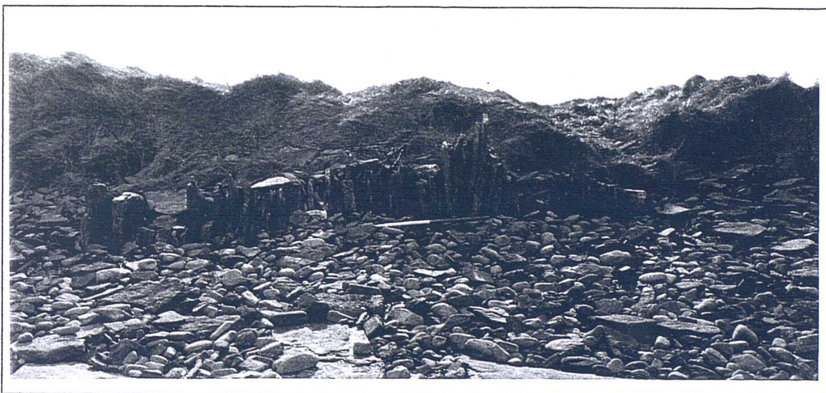
Figure 13 Sea wall construction, Skennist, Papa Westray (Photo: author)
