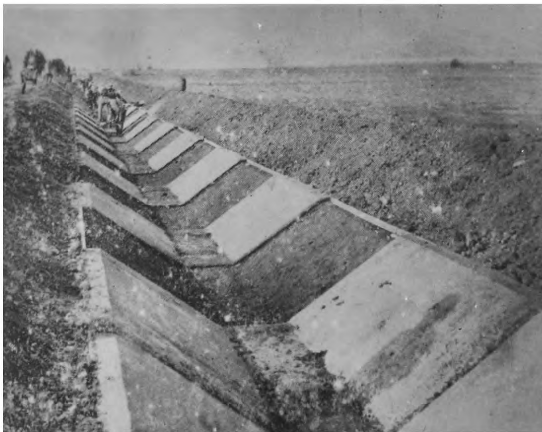
Plate XVI. Lining operations on laterals.
