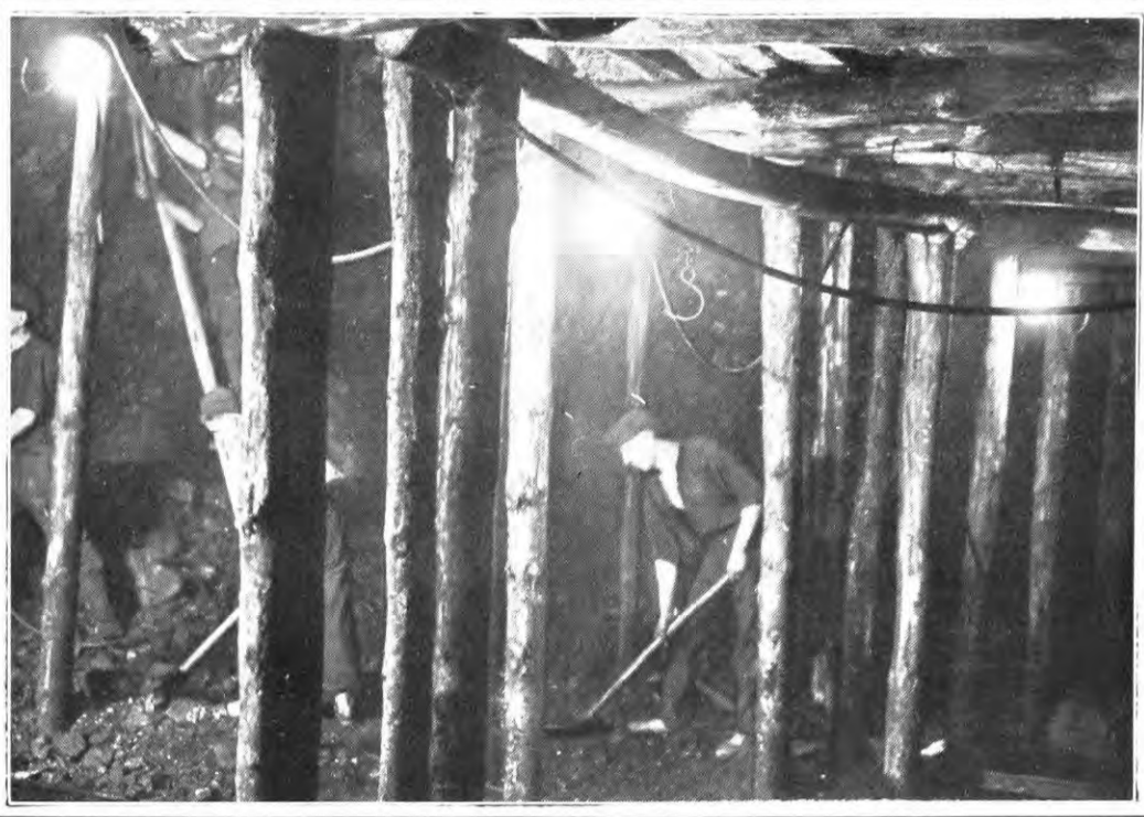
— THE COAL FACE - ROOF SUPPORTED BY WOOD —
