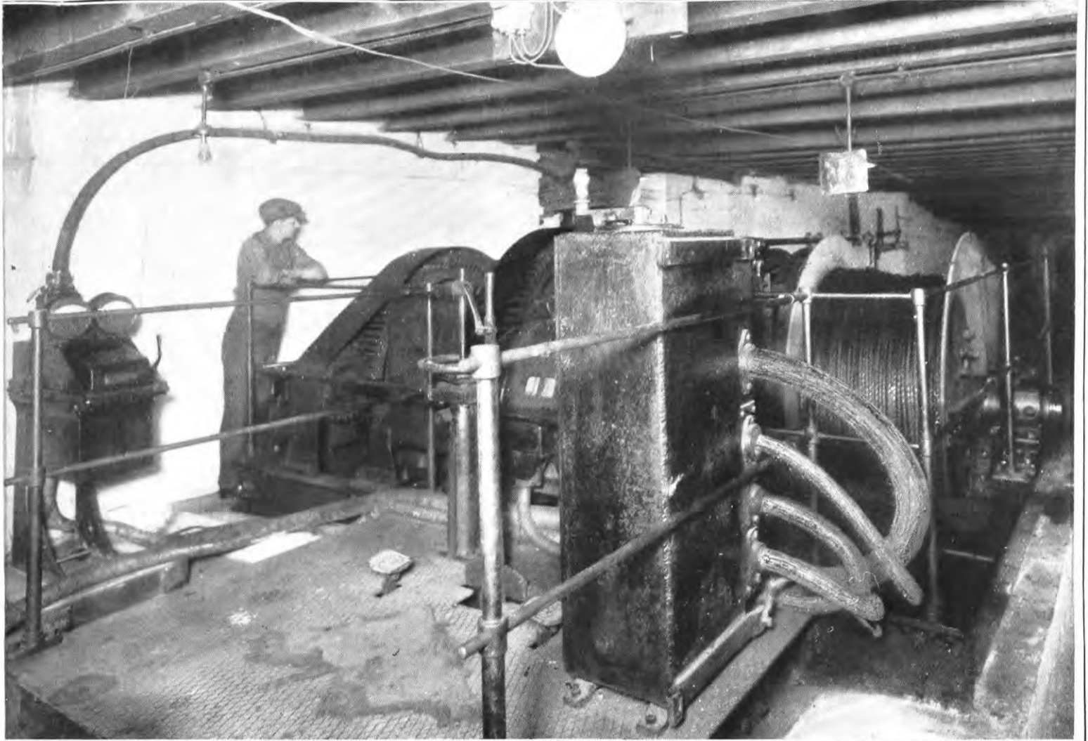
375 H.P. MAIN AND TAIL ROPE HAULAGE.
