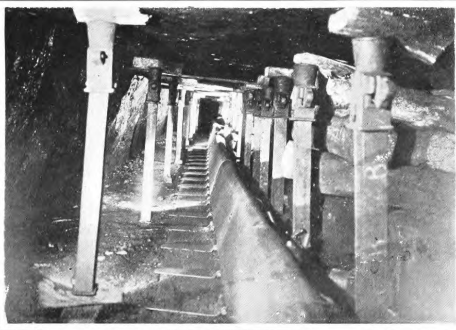
THE COAL FACE - ROOF SUPPORTED BY STEEL.
