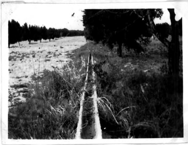
Concrete ditches are practically confined to Italian farms, Oliveti.
