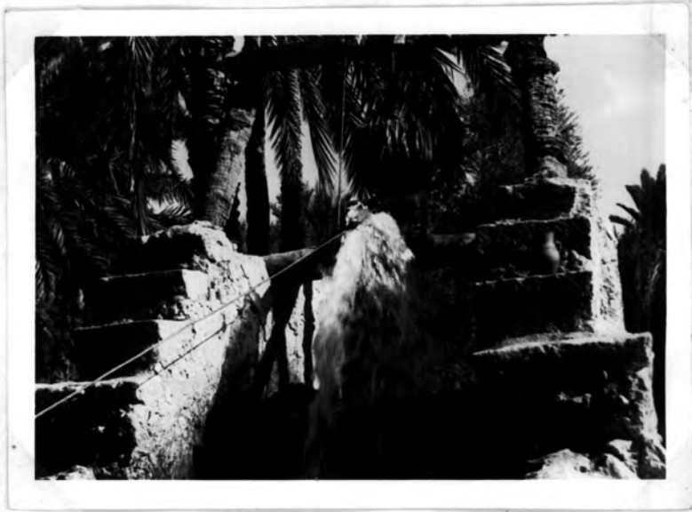
The Dalu, the water lifting bag, Zavia.
