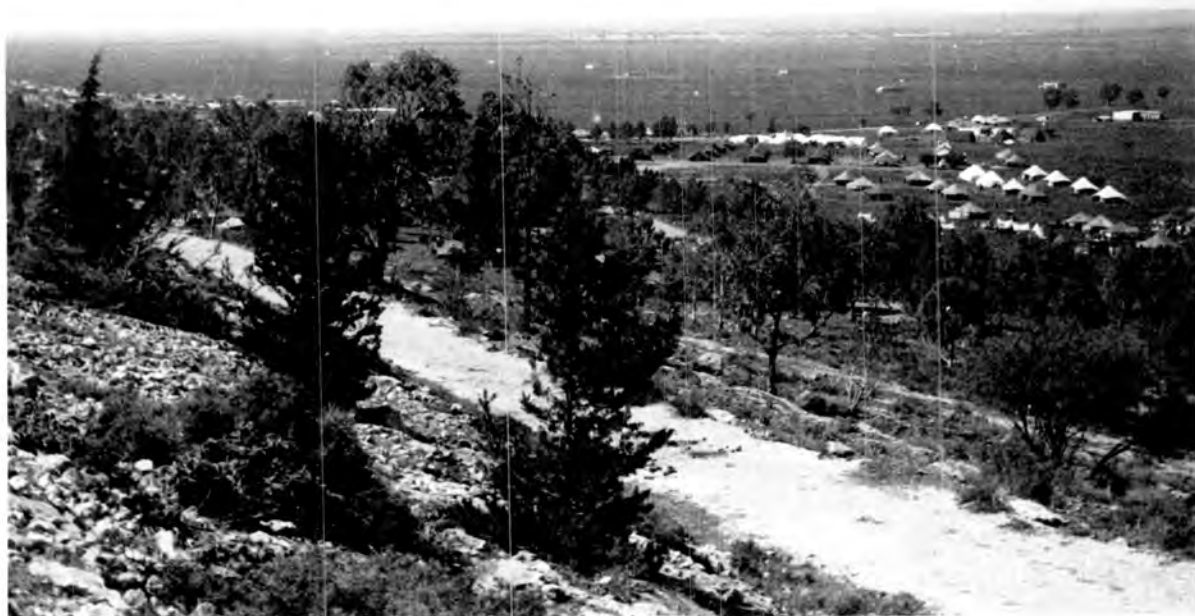
Plate 19 (A) - The refugee camp at the foot of the second escarpment south of El-Marj town. The camp was erected after the earthquake destroyed most of the town.
