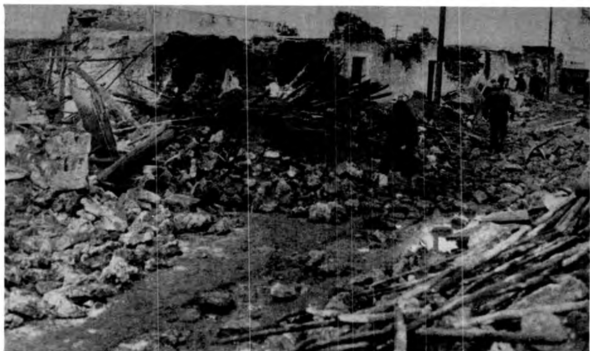
Plate 21 (A) - The heap of rubble stones in Mahallah Esh-Sharqia. The remains of the fallen roof consisting of wooden rafters. Note the houses of rubble stones with Terra Rossa.
