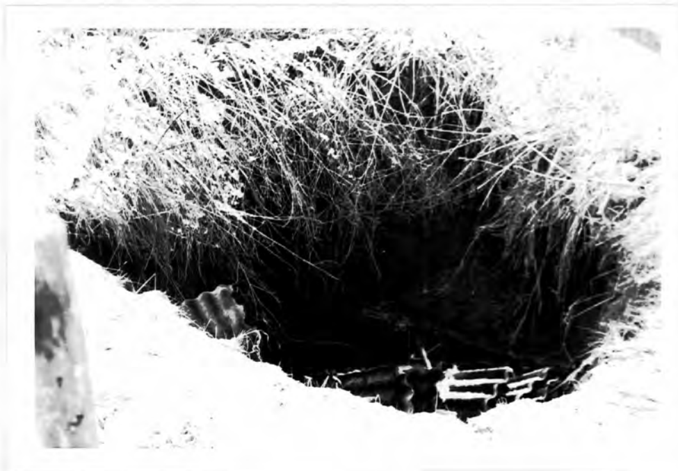
Fig.12. SHAFT KB3. This was probably the shaft worked by the second beam from the engine. It was visible only as an inexplicable diversion in the fence until it caved in in November 1968. It has since been refilled.
